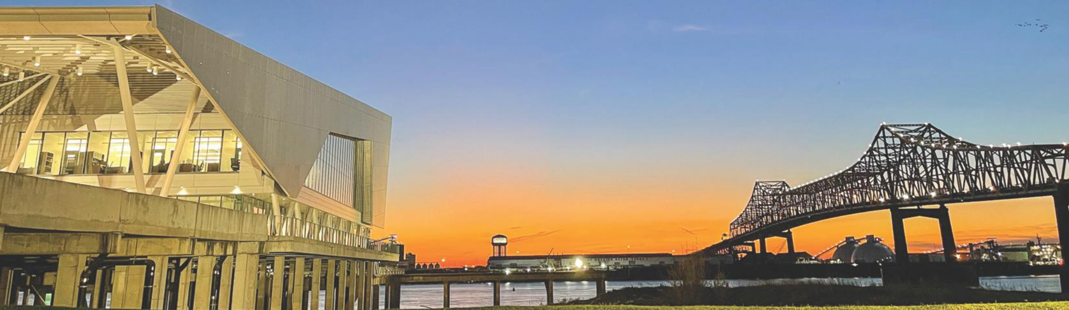
Pictured: The Center for Coastal and Deltaic Solutions (left) & The Mississippi River Bridge
